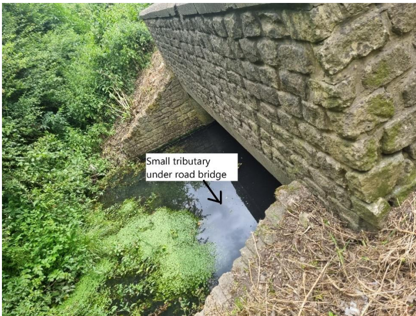
Figure 1.3: Road bridge along the A4095
